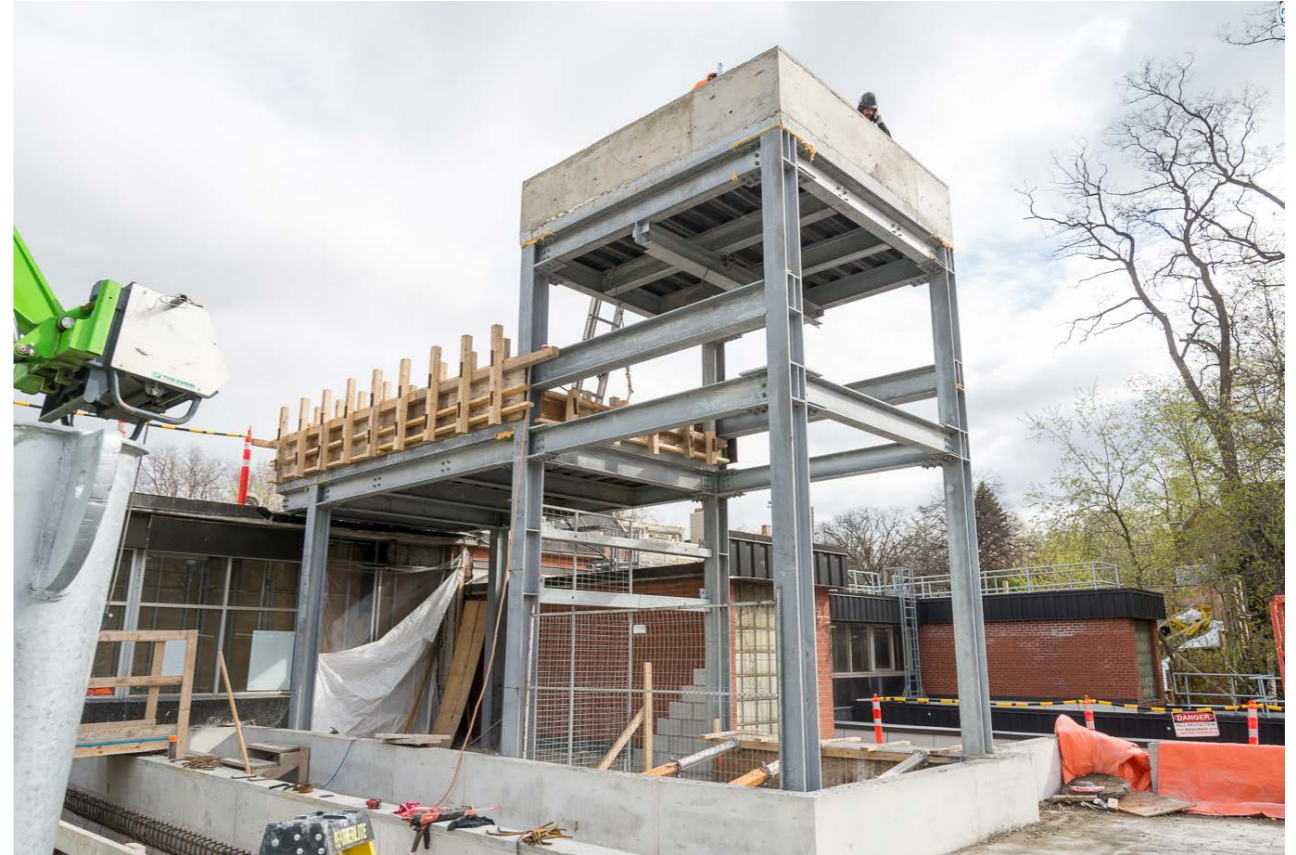
Elevator shaft construction (for southbound), Rosedale Station.
