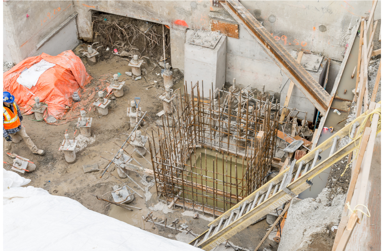
Elevator pit (for northbound), Rosedale Station.
