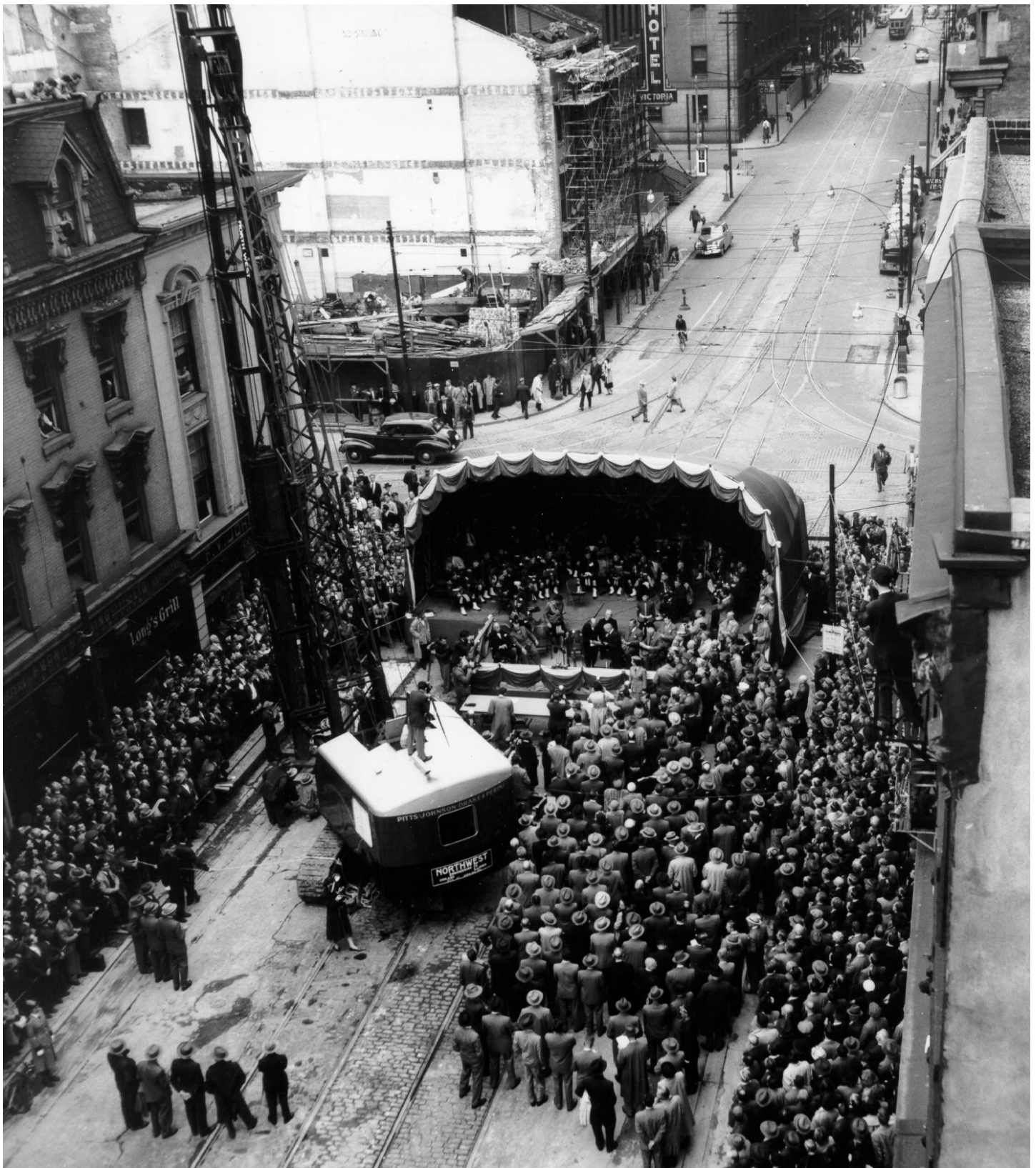
Above: On September 8, 1949: Construction began on the Yonge project, a 4.6-mile subway running under Yonge Street from Front Street to Eglinton Avenue. Construction comprised of 3.2 miles of cut-and-cover and 1.4 miles of open cut.
