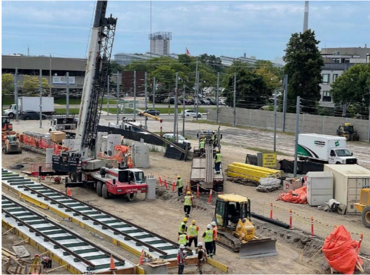
Russell Yard track overhaul
