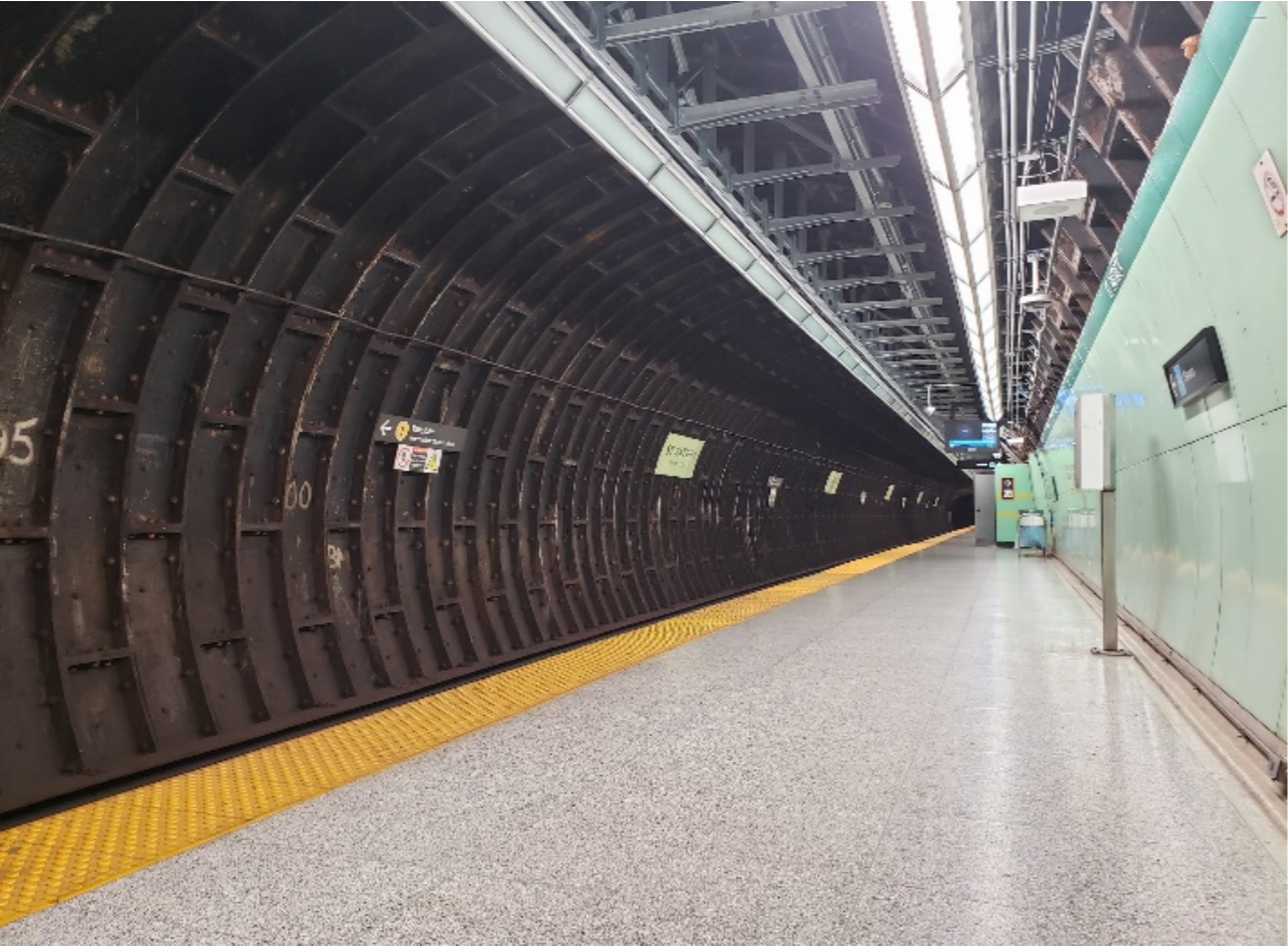
New light fixture installation
