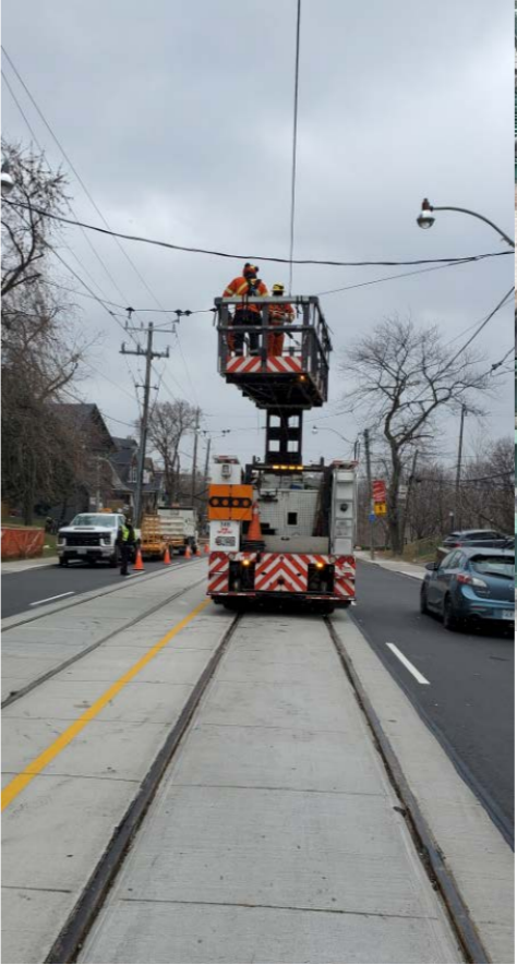
Broadview (Danforth to Gerrard) wire replacement; tangent track replacement
