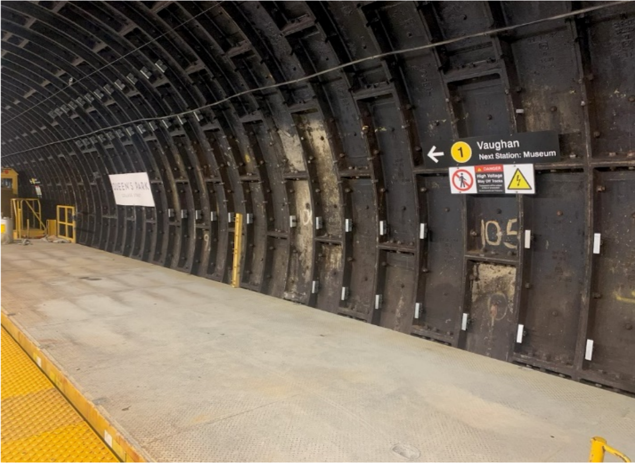
Installation of upper and middle L-brackets
