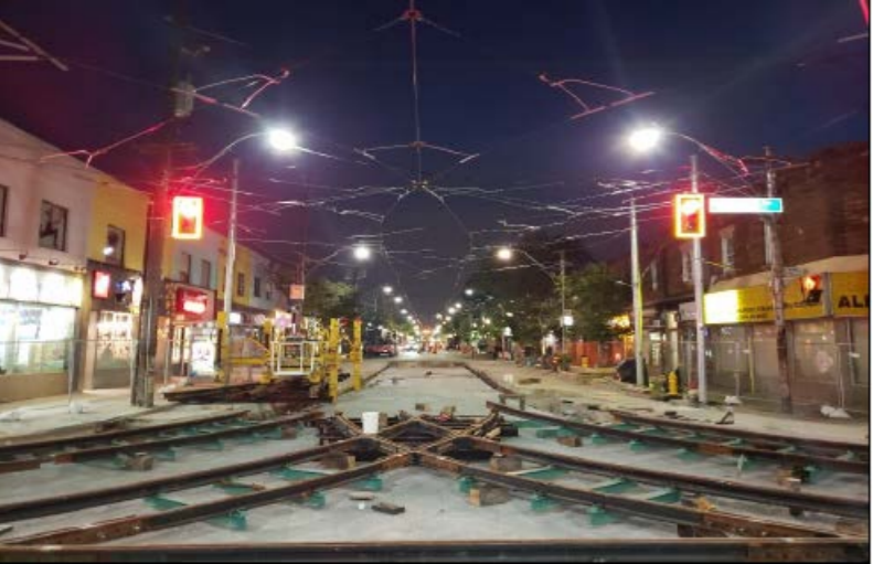
Gerrard and Coxwell intersection track replacement
