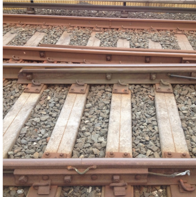
Traditional Wood Ties vs New Composite Ties
