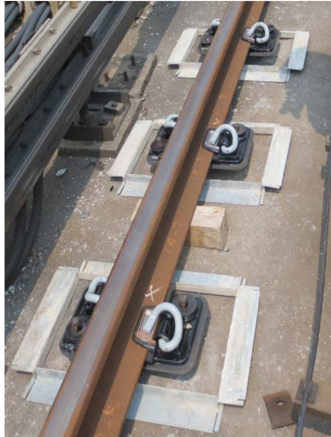
Running Rail Grout Pad
