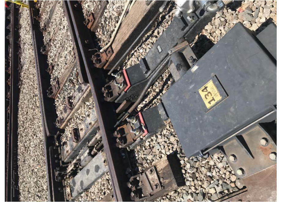
Traditional Wood Ties vs New Composite Ties
