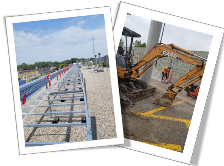
Breaking ground at Birchmount Garage
