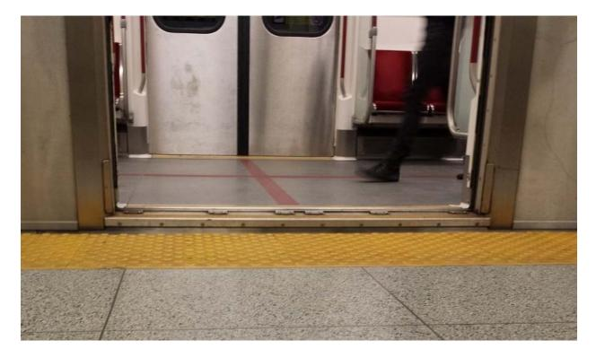
Photo 3a – Pre-existing vertical gap at Eglinton Station.
