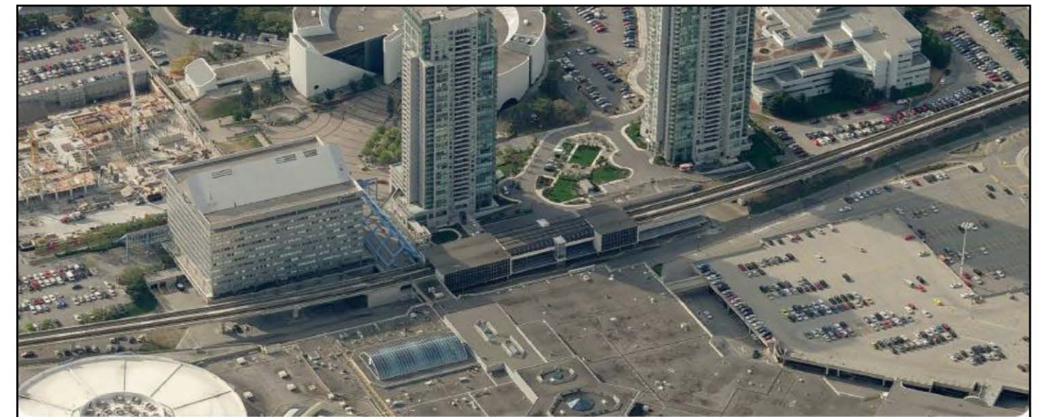
Exhibit 2-10: Existing Scarborough Centre Station, looking south
