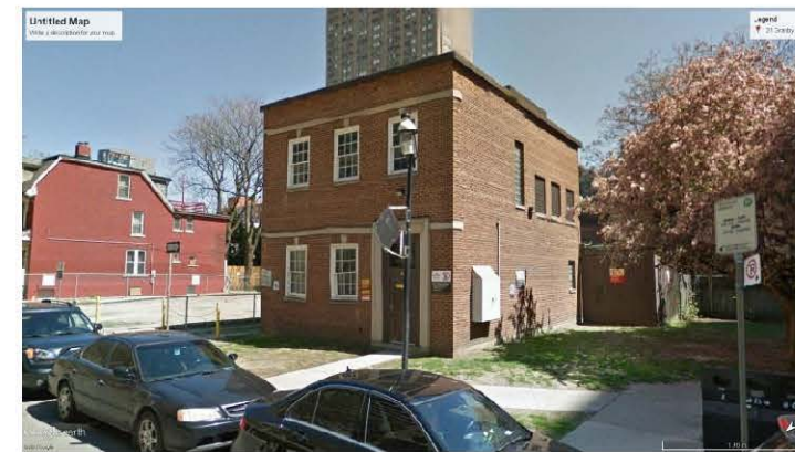
Exhibit E4-5: Traction Power Substation – 21 Granby Street, Toronto
