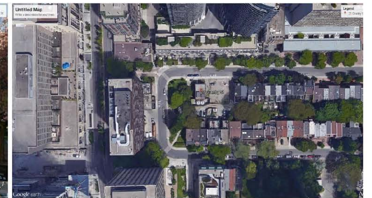
Exhibit E4-6: Traction Power Substation – Aerial View
