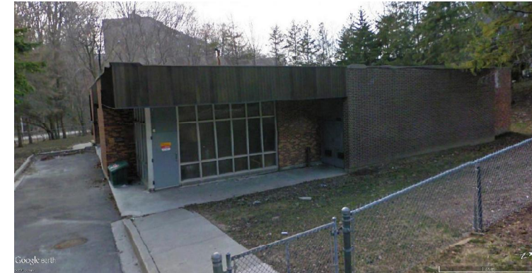
Substation at 4 Glenayr Rd. on Line 1 between St. Clair West Station and Eglinton West Station
