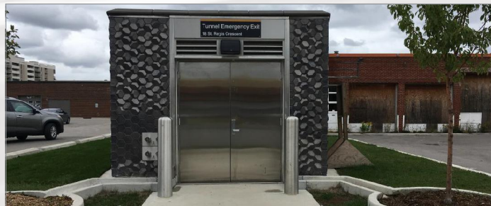
Emergency Exit Building
