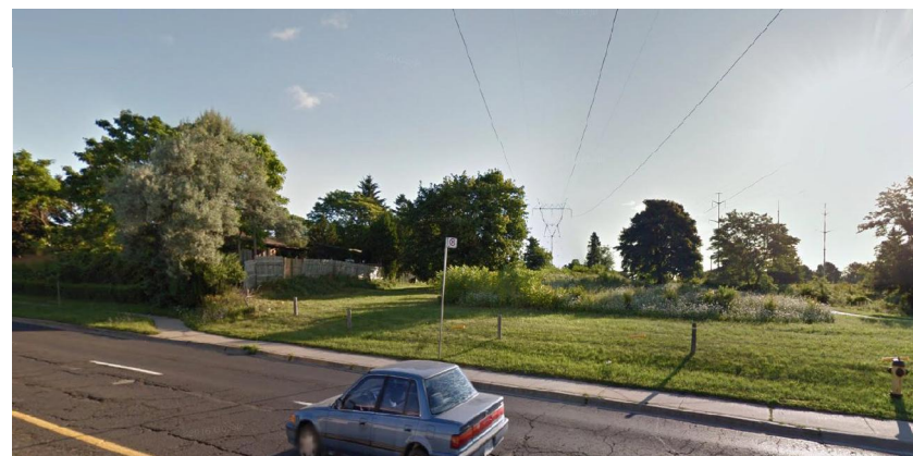
South limit of substation zone under live power lines
