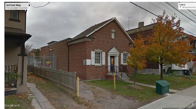
587 Lansdowne Ave. on Line 2 near Lansdowne Station
