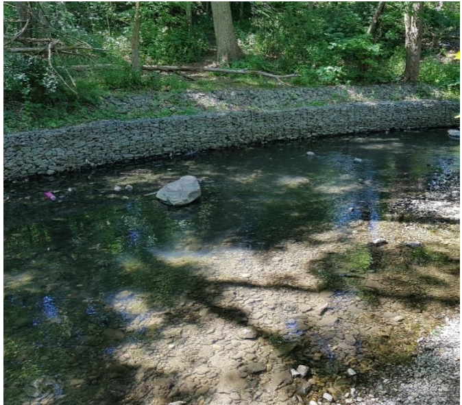
Photograph 12 ↑ Reach 2 Gabion baskets along the left bank, looking upstream
