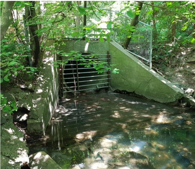
Photograph 19 ↑ Reach 3 Inlet/outlet northern extent of survey, looking upstream
