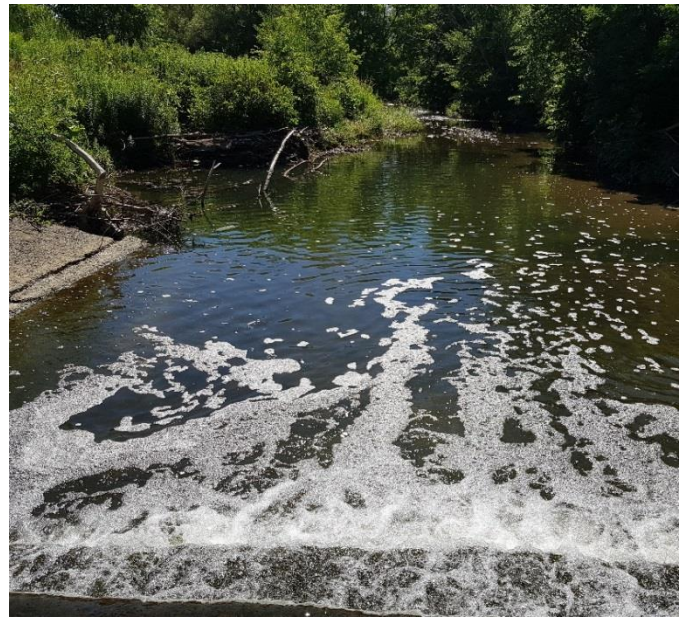
Photograph 8 ↑ Reach 1 Concrete step dam, looking downstream towards the McCowan Road bridge
