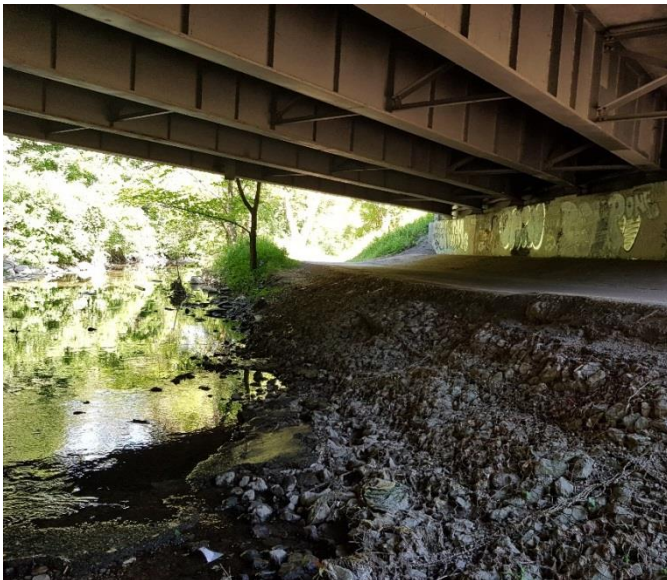
Photograph 3 ↑ Reach 1 Gabion baskets under McCowan Road bridge, right bank
