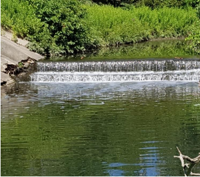
Photograph 9 ↑ Reach 1 Concrete step dam, looking upstream towards Legion Road
