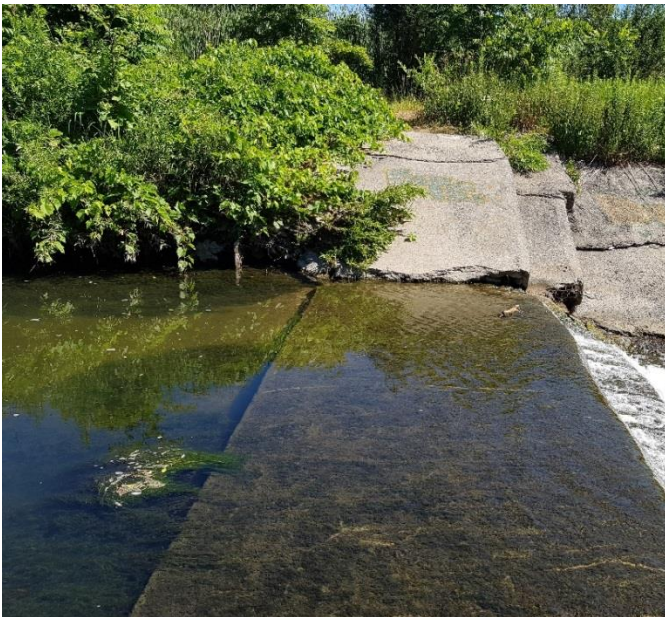
Photograph 7 ↑ Reach 1 Concrete step dam, looking towards the right bank (east)
