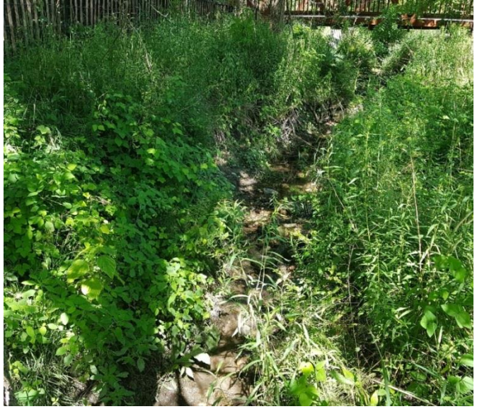
Photograph 10 ↑ Reach 2 West Highland Creek tributary dry, looking north
