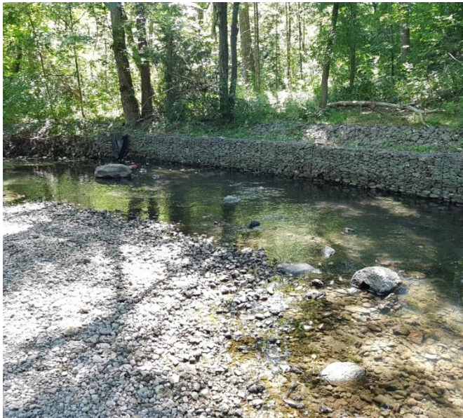
Photograph 15 ↑ Reach 2 Gabion baskets along the left bank with increased cobble in the channel, looking downstream
