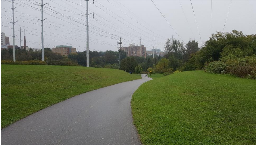
Photo 6: Overview of the disturbance within the Gatineau Hydro Corridor, west of McCowan Road; view southwest
