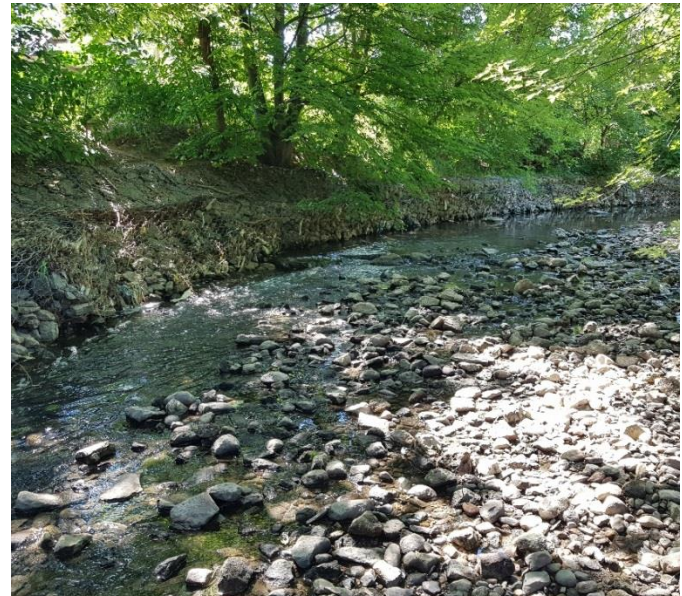
Photograph 16 ↑ Reach 2 Gabion baskets along the left bank with increased cobble in the channel, looking upstream
