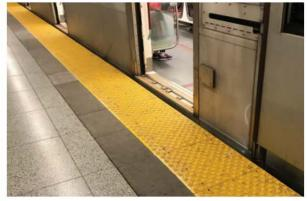
If you've travelled through Eglinton Station, you may have noticed some new, sloped platform edge tiles. The tiles are designed to reduce the vertical gap between the train and the platform edge as part of an effort to improve barrierfree access across the TTC's network. Please be mindful of the new platform edge and as always, be careful boarding and disembarking from the train.
