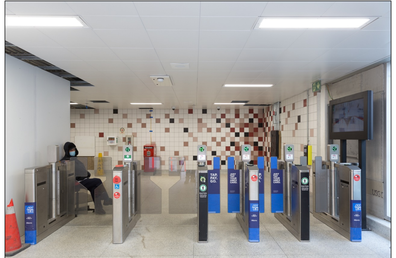
Picture- The fare gates by the new main entrance at Summerhill Station
