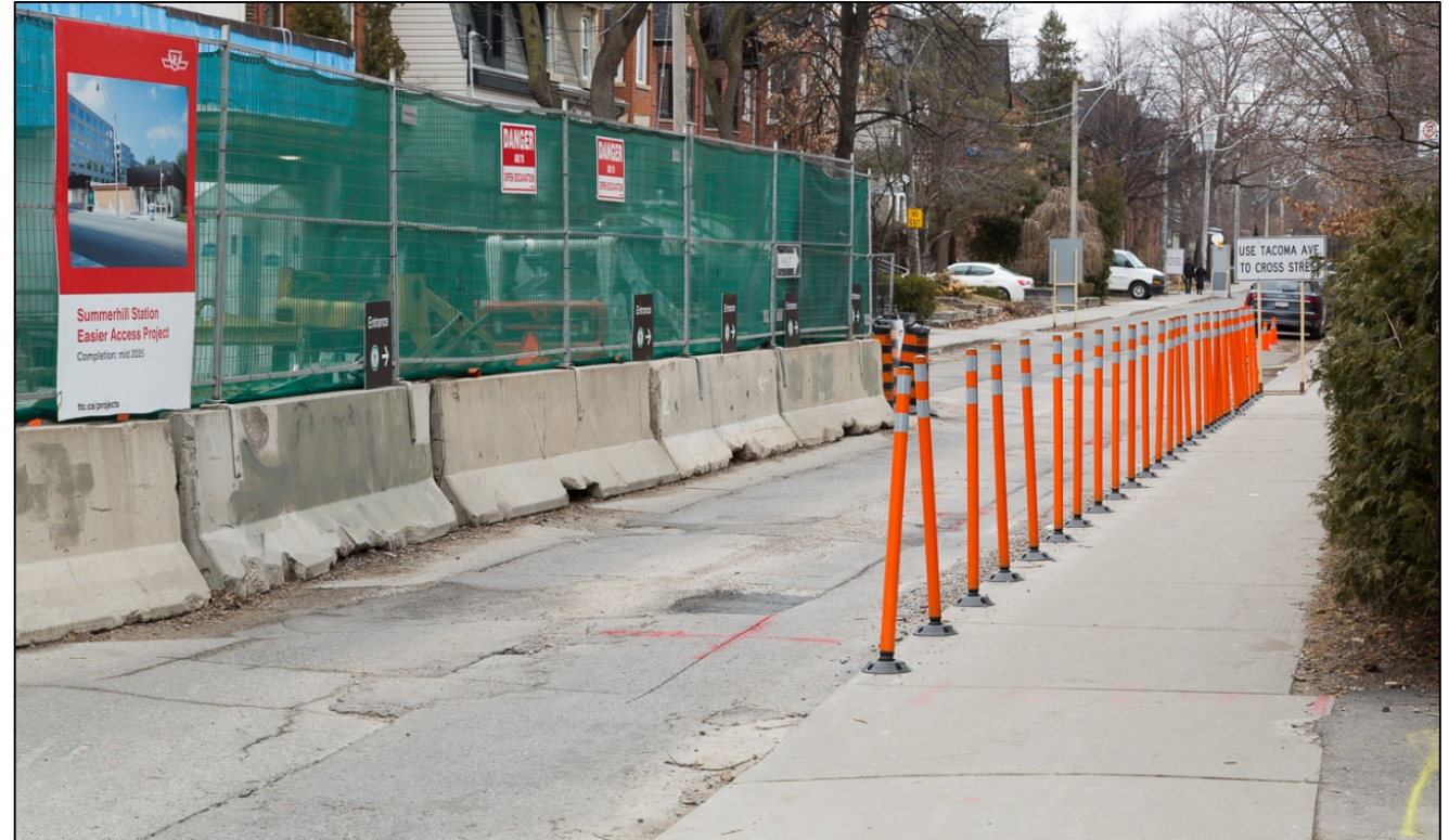
Picture- Outside the construction site on Shaftesbury Avenue
