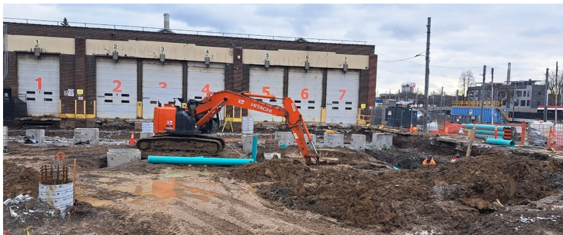
Concrete and track work removal and excavation
