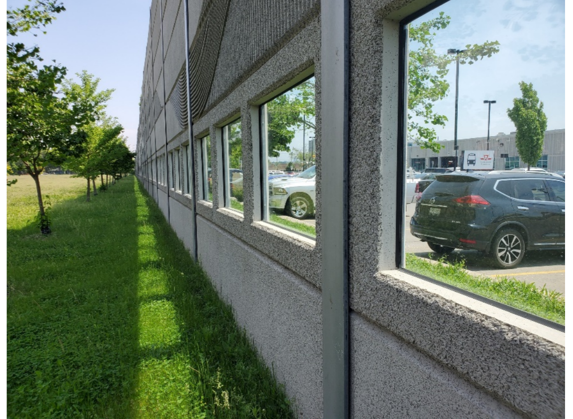
Current Mount Dennis Garage parking lot with noise wall. Noise wall to remain.
