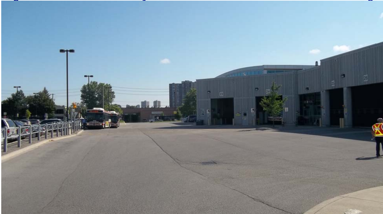
Figure 2-1: A View of the Bays at the North End of Mount Dennis Bus Garage
