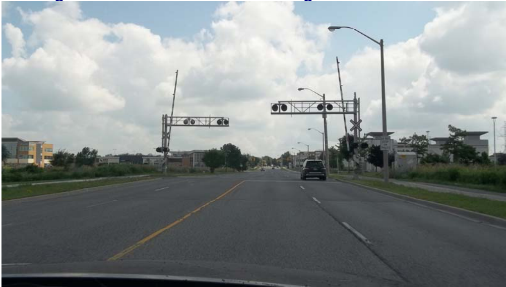
Figure 4-2: At-Grade Rail Crossing at McNicoll Avenue
