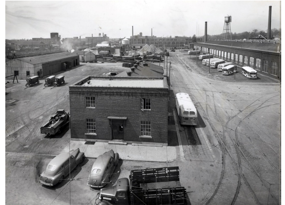
Hillcrest Complex looking west (1944).
