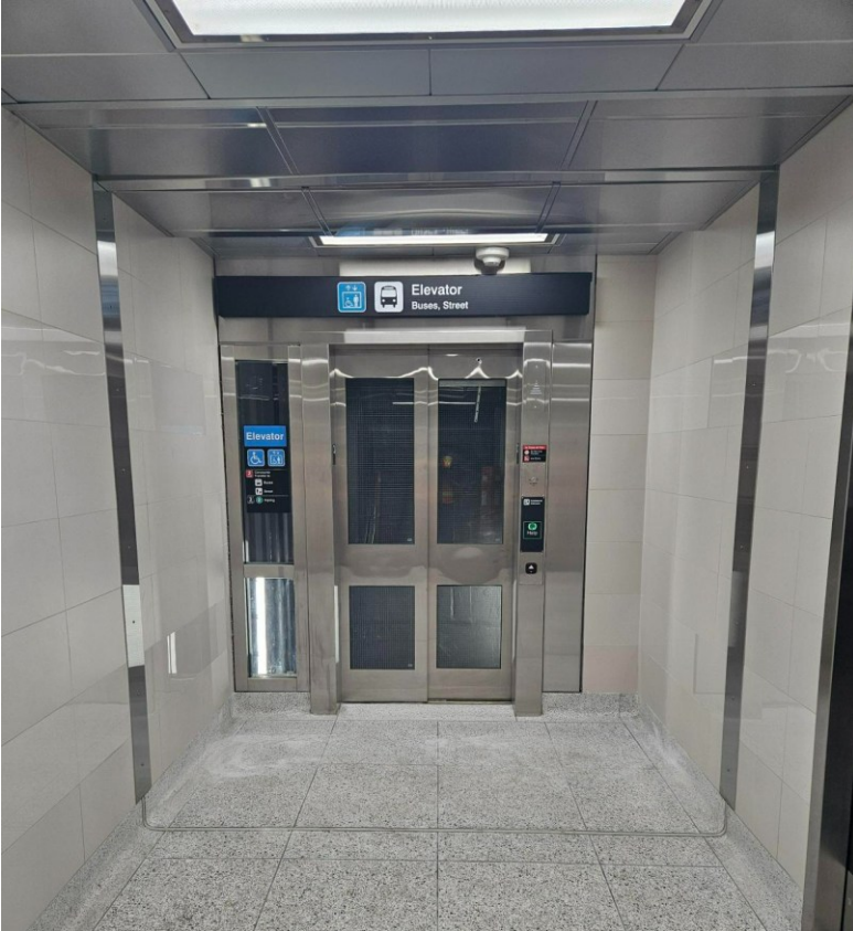
Photo: Elevator 1 (E1) Platform level - Eastbound
