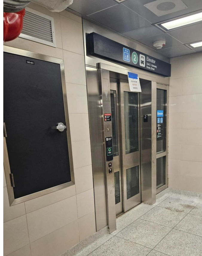
Photo: Elevator 1 (E1) Concourse level - Eastbound
