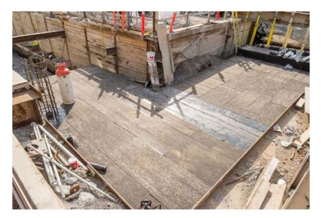
Photo- Looking southeast at waterproofing of the Dewhurst passageway and the westbound platform access roof
