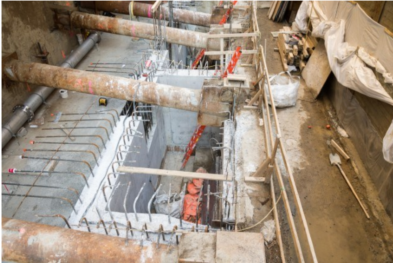
Photo of: North side/end elevator pit wall for slab to be poured on top of with concrete.
