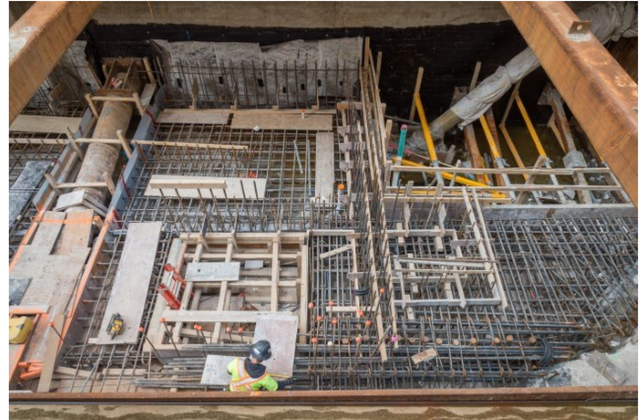
Photo of: Formwork and rebar around elevator pit – to be poured with concrete.
