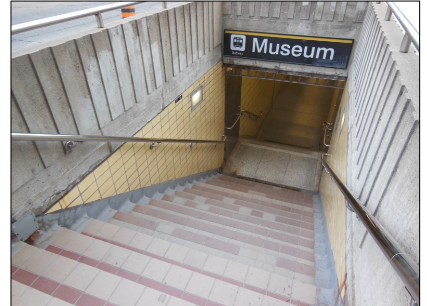
Existing stairway entrance/exit at Museum Station
