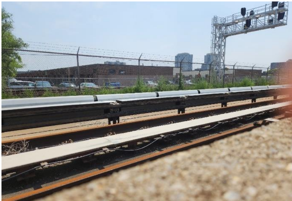
Image 17: TTC existing Line 3 tracks between Ellesmere and Lawrence Stations, facing south.
