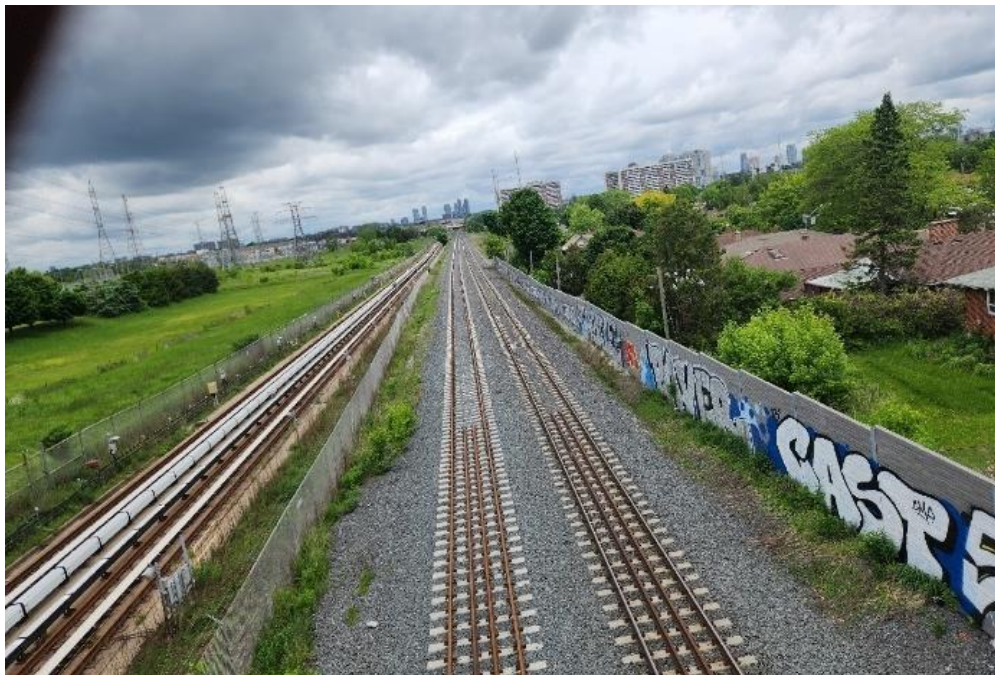
Image 4: TTC existing Line 3 tracks south of proposed Tara Avenue Station, facing south.
