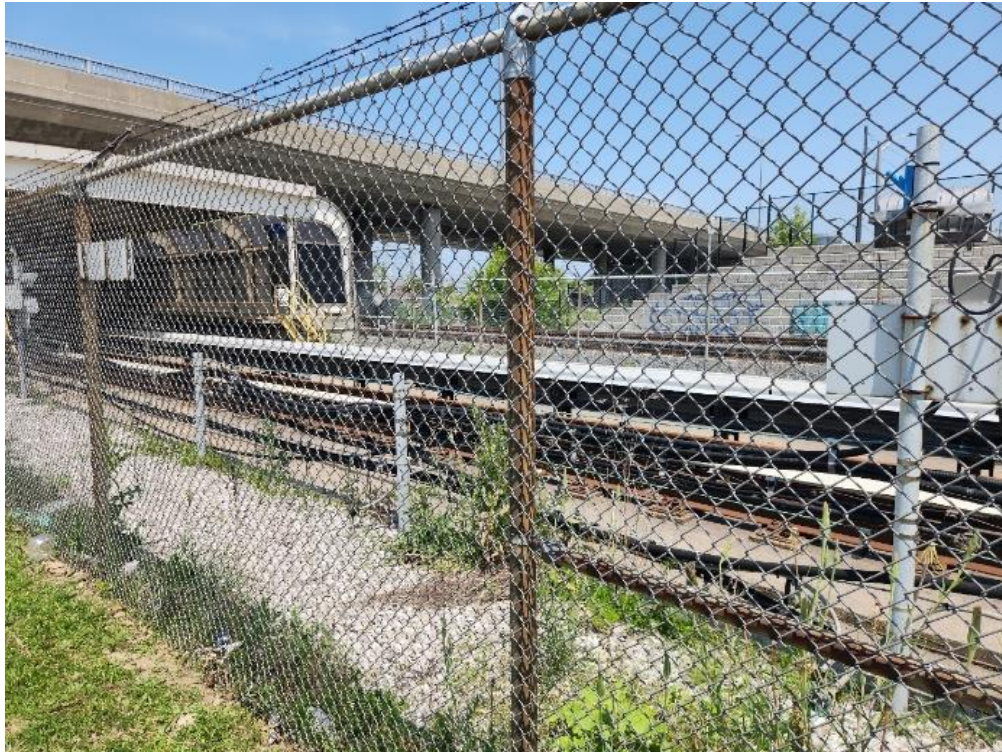
Image 23: TTC existing Line 3 tracks, facing northeast.
