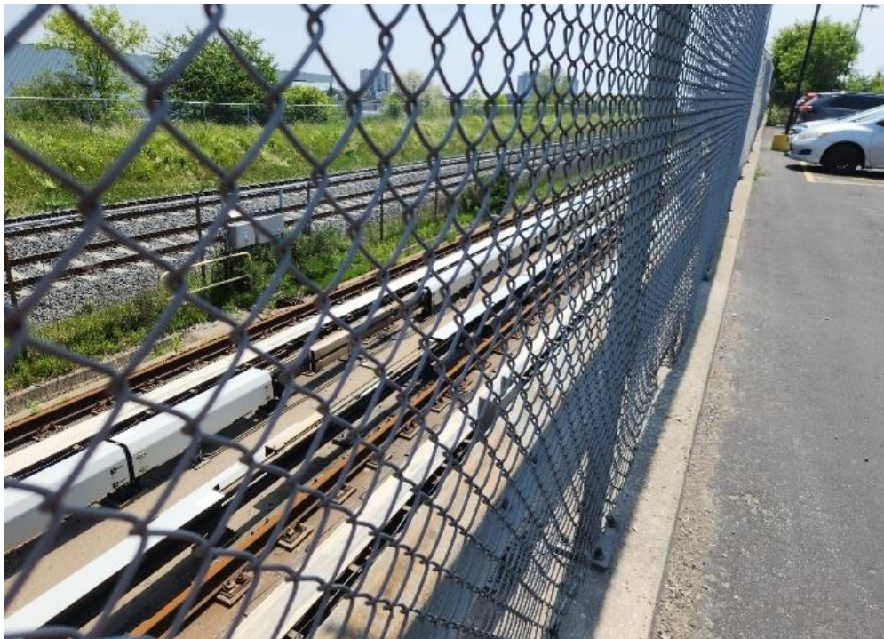
Image 19: TTC existing Line 3 tracks between Ellesmere and Lawrence Stations, facing south.
