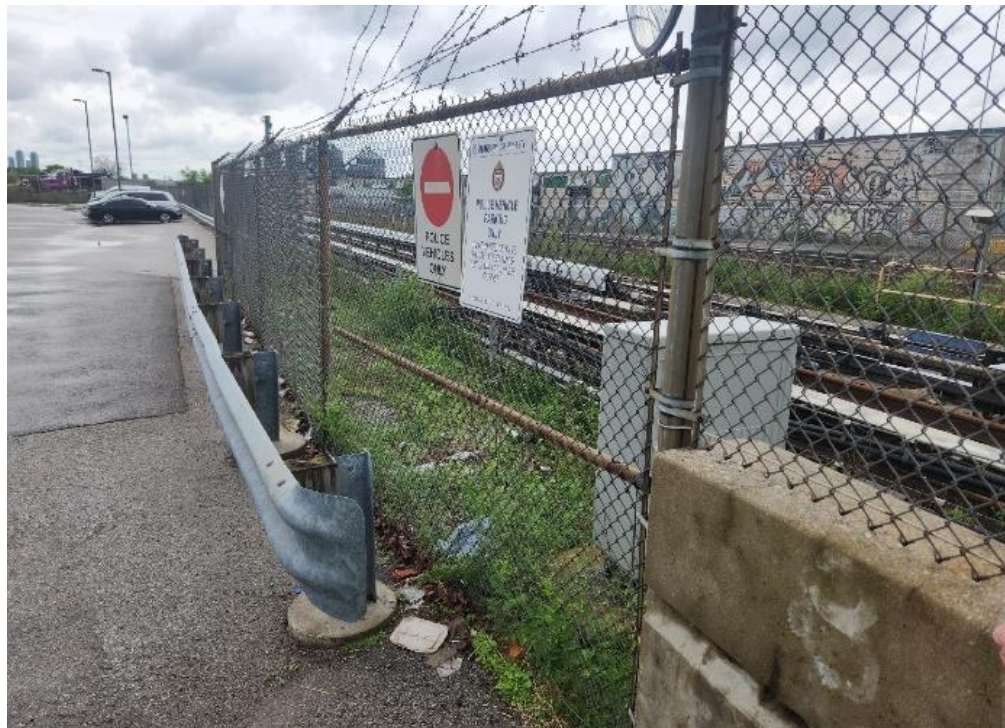
Image 15: TTC tracks directly north of Lawrence East Station, facing north.
