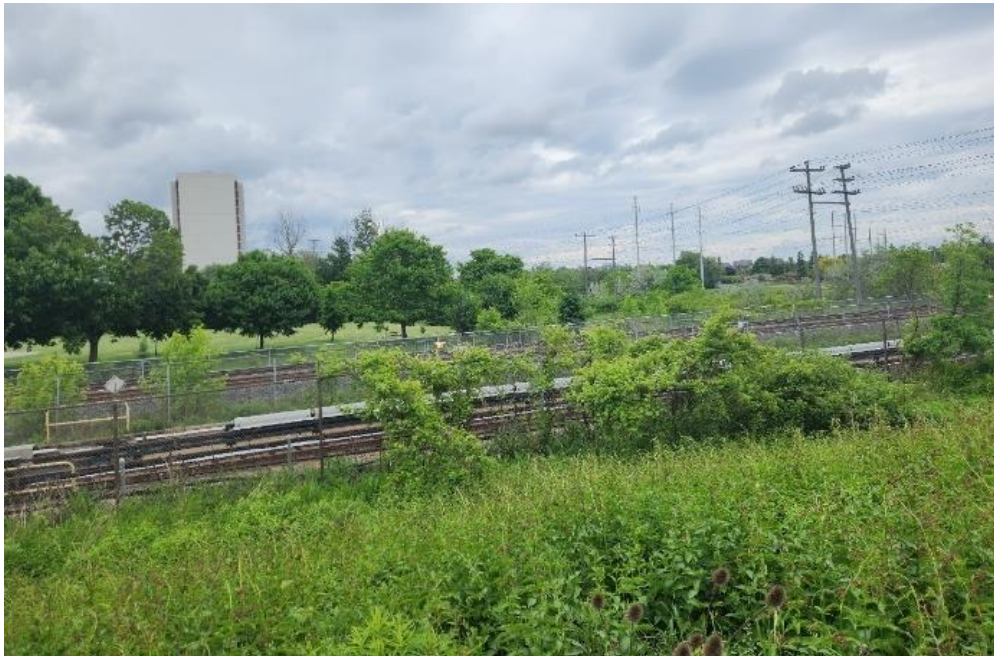
Image 11: TTC existing Line 3 tracks between Lawrence Station and Tara Avenue, facing east.
