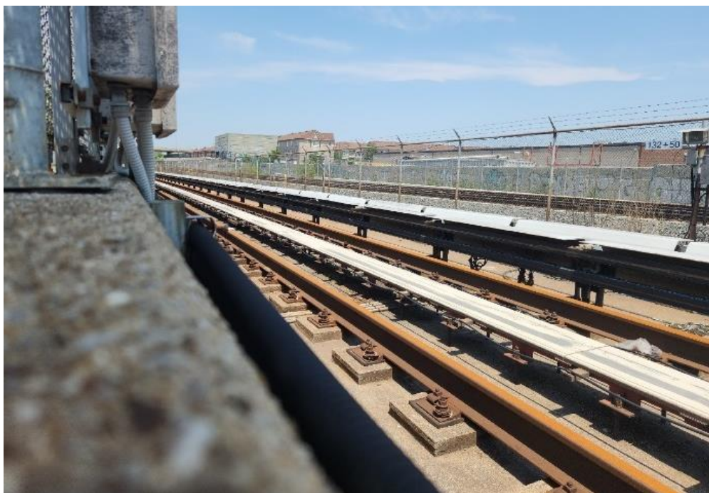
Image 20: TTC existing Line 3 tracks south of Ellesmere station, facing north.
