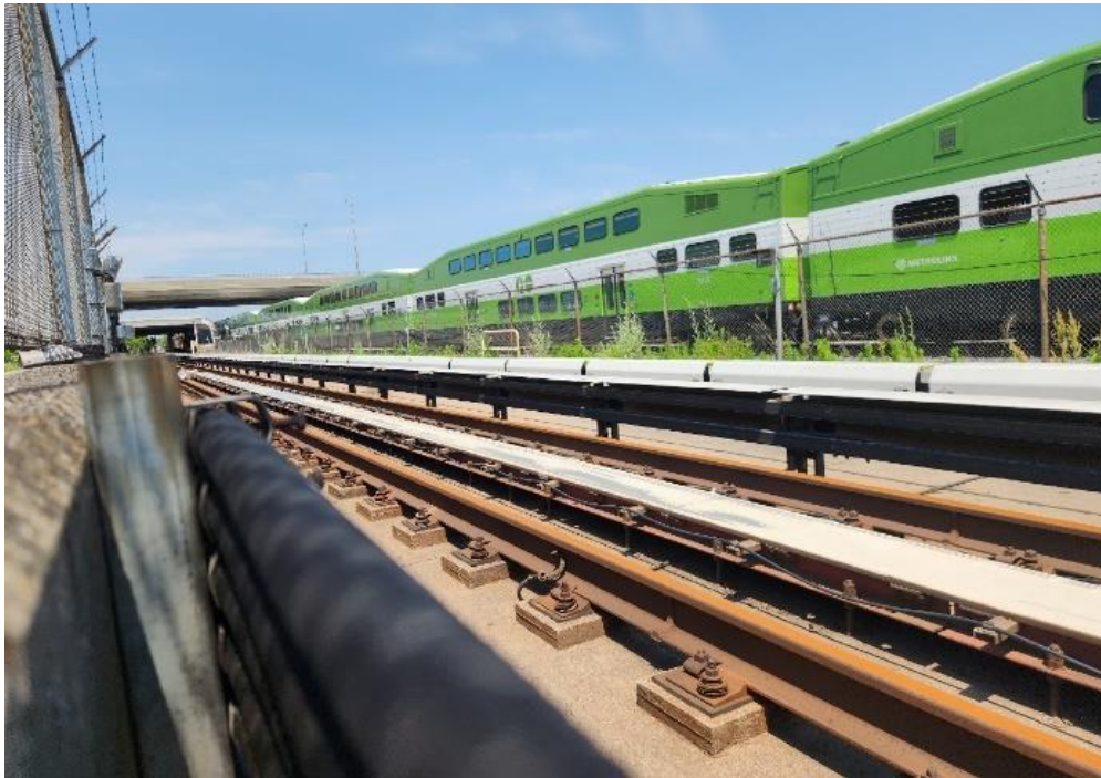
Image 21: TTC existing Line 3 tracks south of Ellesmere station, facing north.
