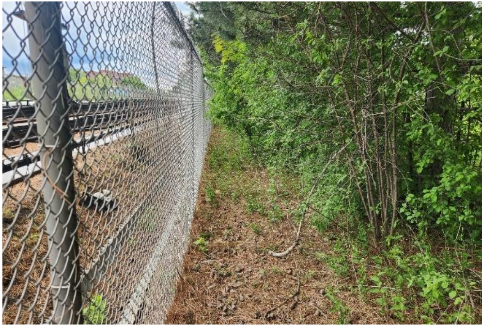
Image 3: TTC existing Line 3 tracks south of proposed Tara Avenue Station, facing southeast.
