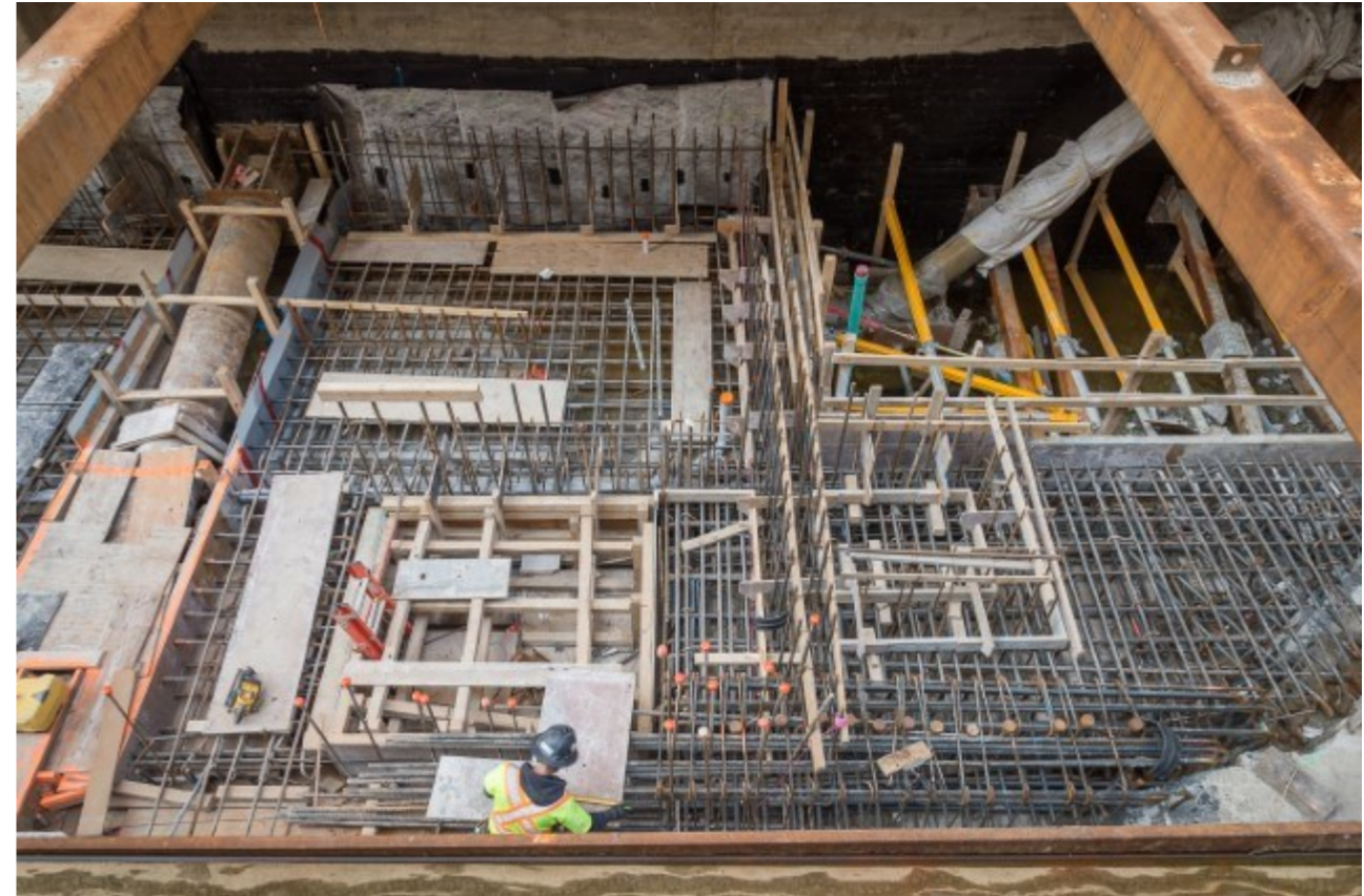
Formwork and rebar around elevator pit – to be poured with concrete.
