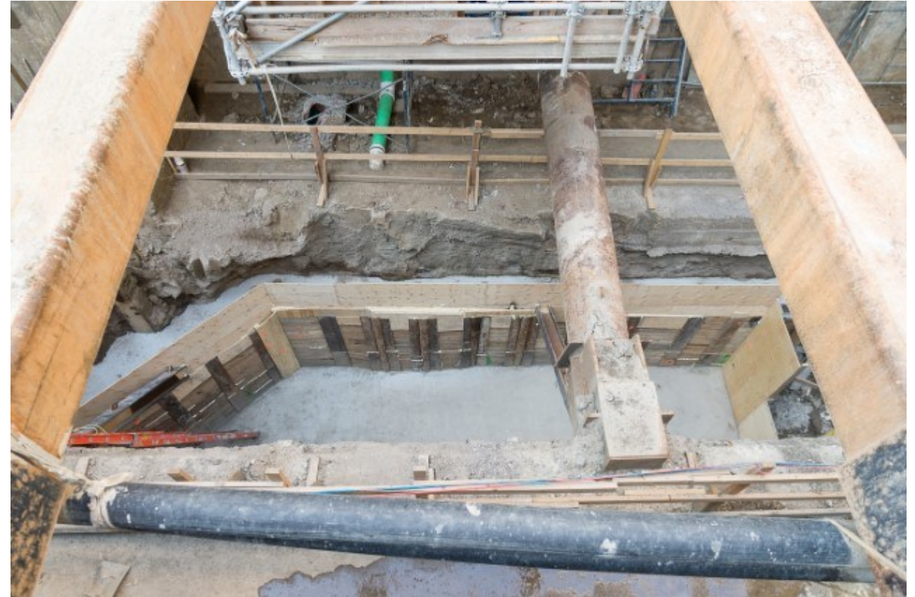
Photo of: Mud slab at the south end excavation to aid in the development of new concourse and stairs from platform level.
