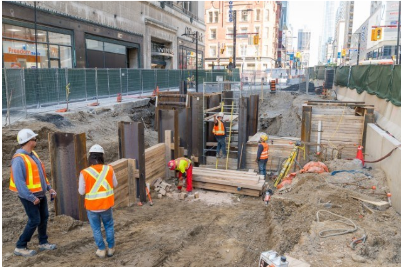
Photo of: Finger piles being placed on the north end of the site, to perform shoring support via timber piles.
