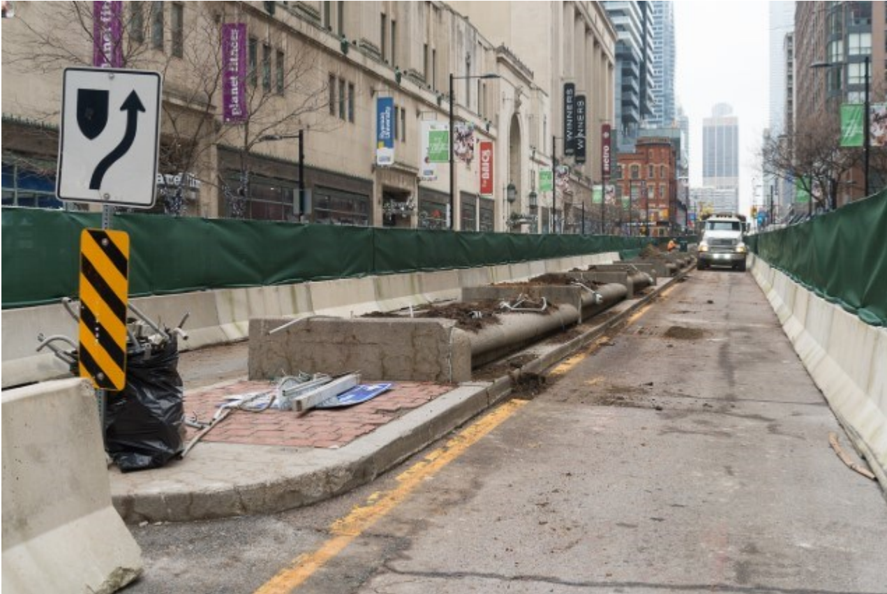
Photo of: Median Demolition – median to be removed down Yonge St. in order to start Stage 2 demolition and excavation.
