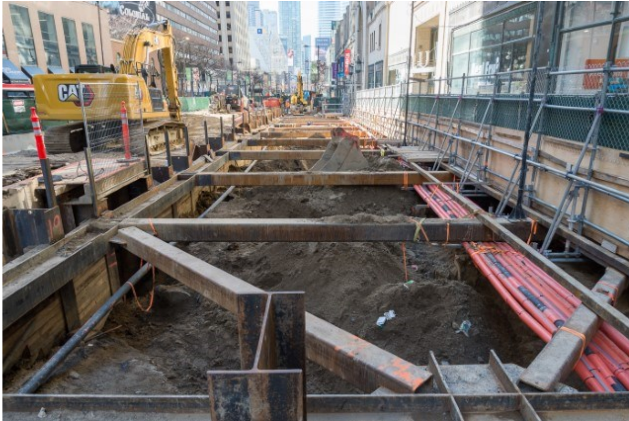
Photo of: Walers, struts and horizontal hollow steel section beams in order to support shoring for further excavation.
