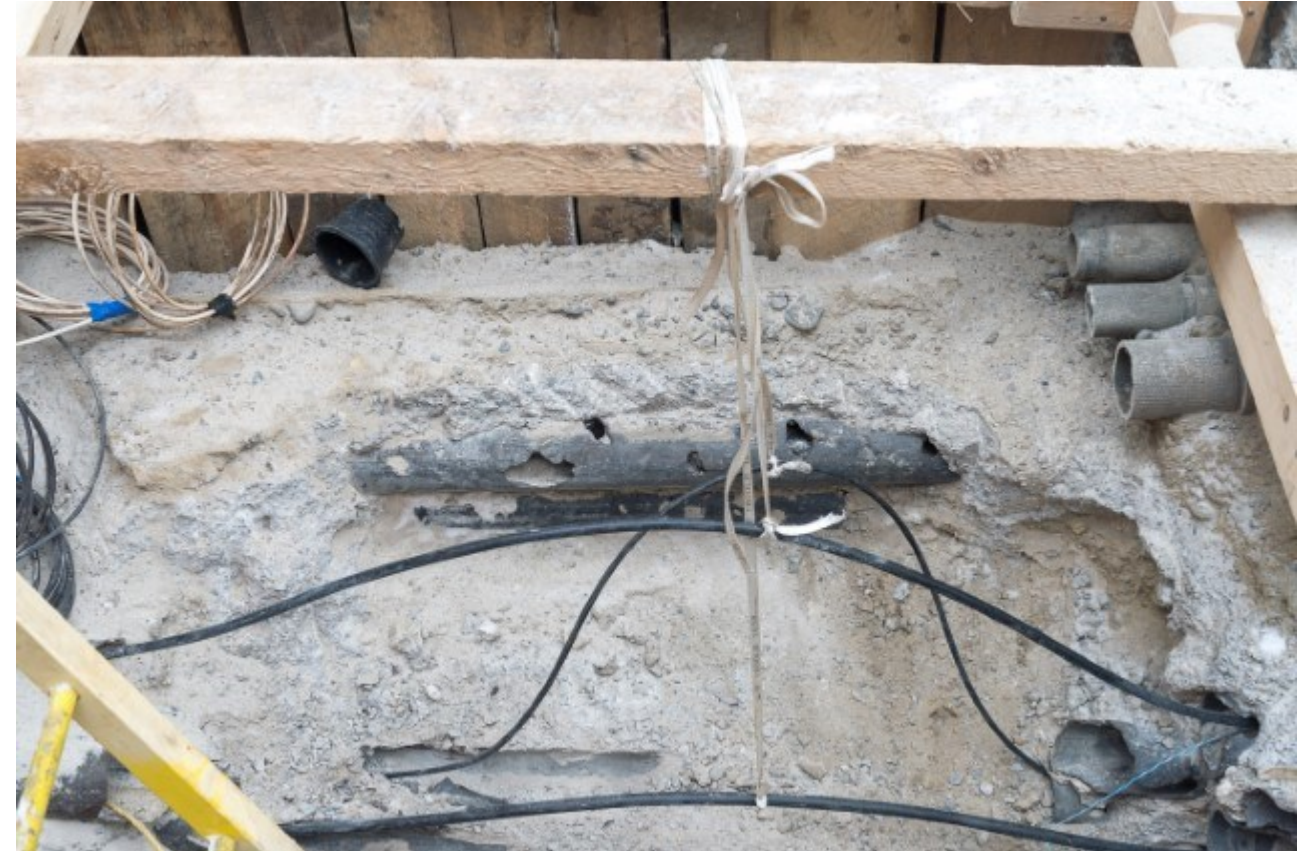
Photo of: Exposed duct banks to be rerouted below ground – exposed conduits to be reattached and fitted with utilities such as telecommunications, internet, electrical etc.
