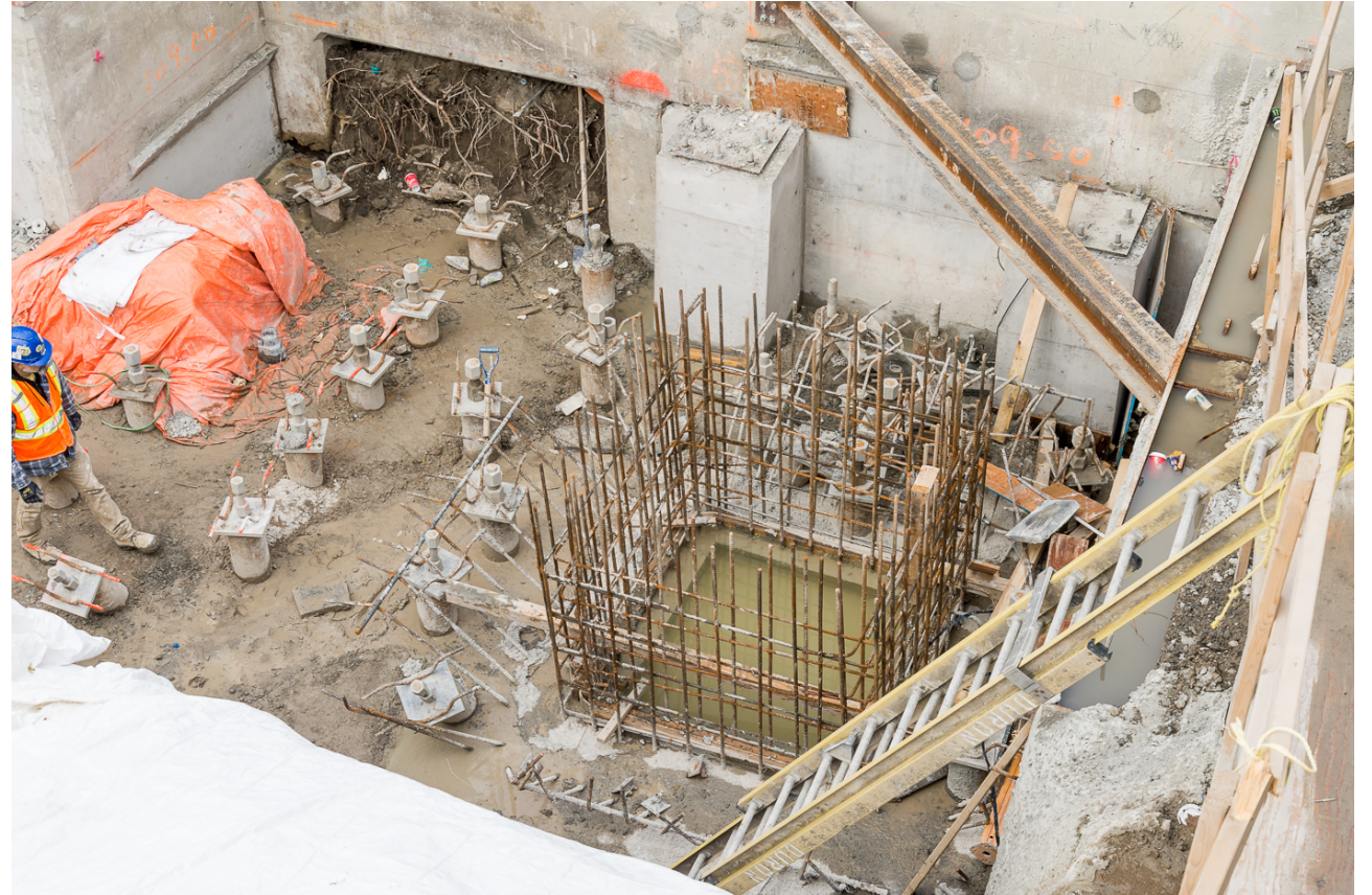
Elevator pit (for northbound), Rosedale Station.
