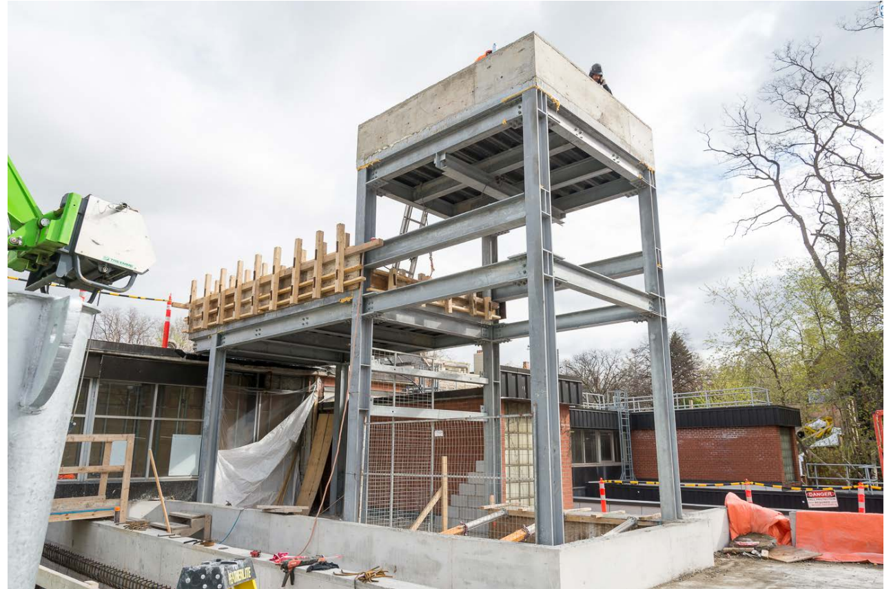
Elevator shaft construction (for southbound), Rosedale Station.
